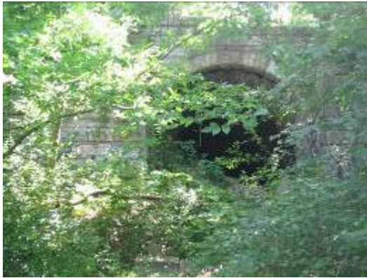
Abandoned Pedestrian Tunnel
